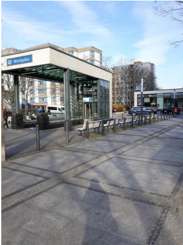
U-Bahn Station Wutzkyallee
